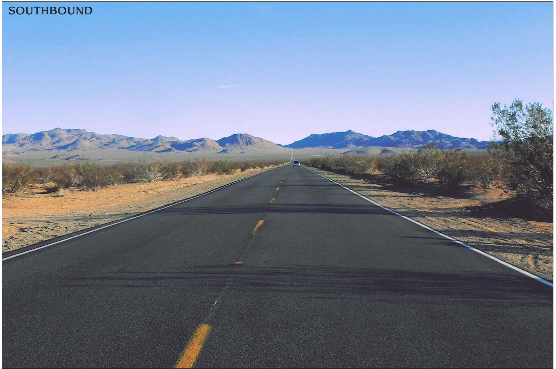
Figure 66S - Scenic View: The southbound traveler enjoys the perfectly straight gently rising highway heading into the Ord Mountains and Goat Pass looking south from PM 66.
