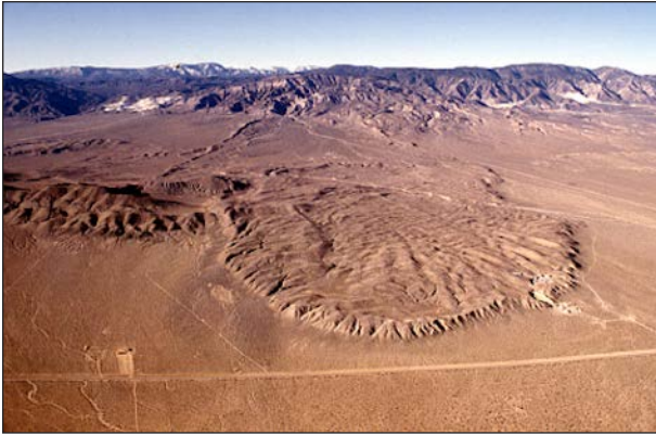
Figure 34A: Aerial view of the Blackhawk Landslide. SR 247 crosses below the slide. Photo by Kerry Sieh
