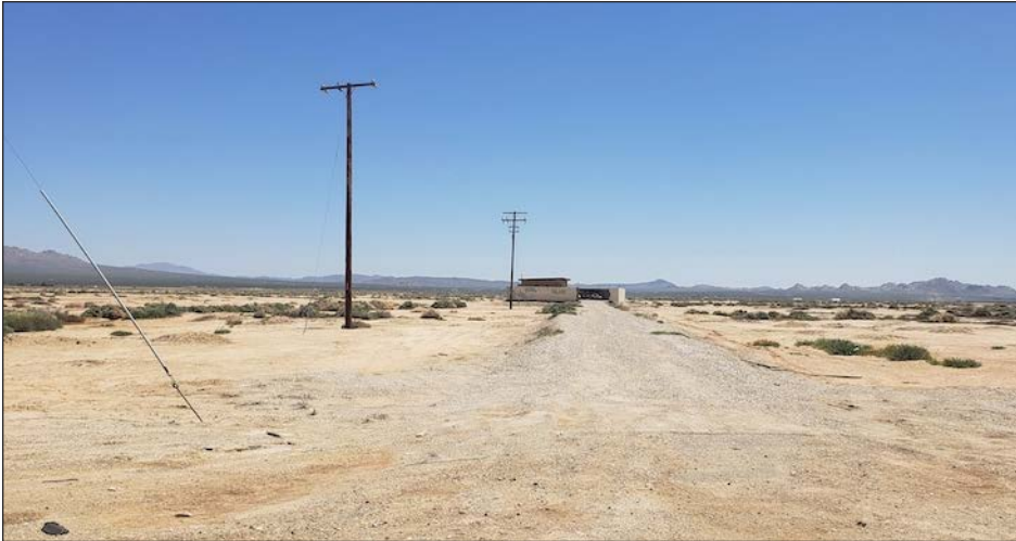
Figure 50.2E - Intrusion: An abandoned radio broadcasting building sits 400' off the highway at PM 50.2 looking east.
