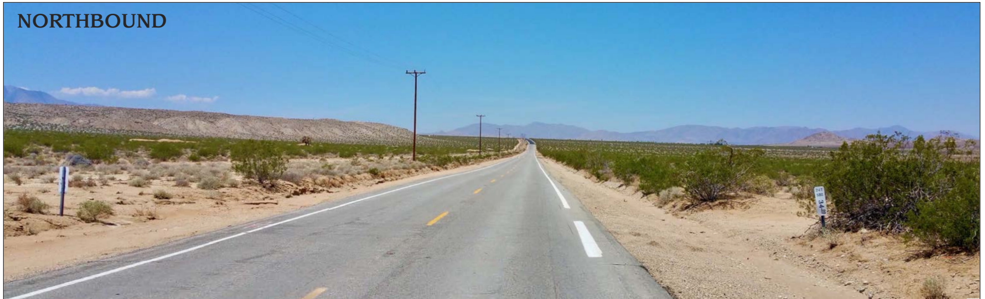
Figure 34W - Scenic View: The Blackhawk Landslide is seen on the left, viewed by the northbound traveler looking west at PM 34. The Granite Mountains are seen straight ahead at a distance of eighteen miles. On the right is Cougar Buttes.
