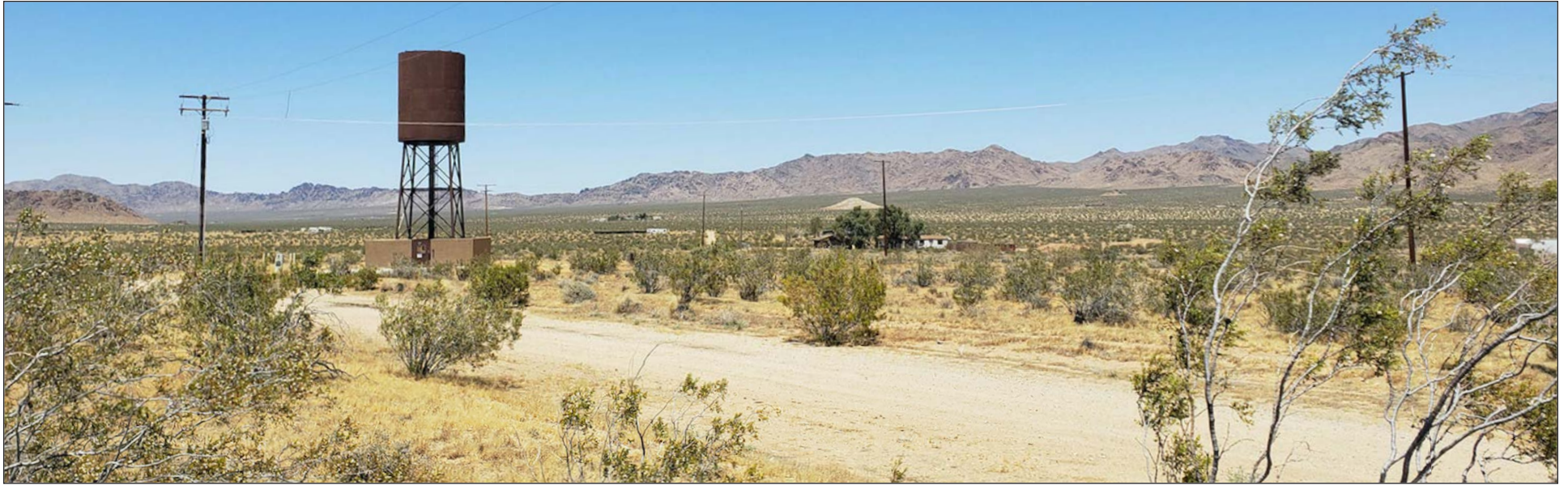
Figure 54.75NE - Intrusion: At PM 54.75 looking northeast is a cell phone tower and structure disguised to look like an old water tank, creating unity with the region.
