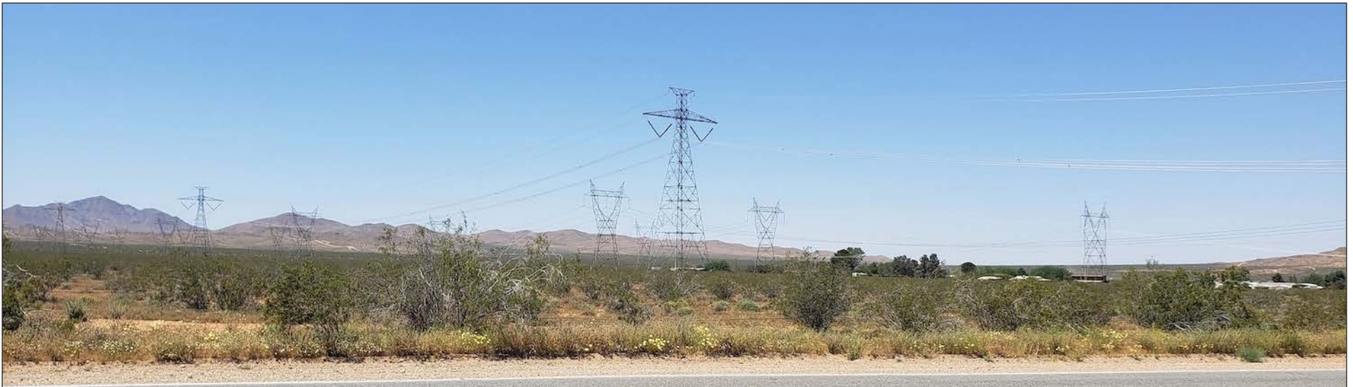
Figure 68.75W - Intrusions: Looking west from PM 68.75, transmission lines dominate the landscape, degrading the scenic view. A neighborhood of homes at Slash X Ranch is seen beyond.
