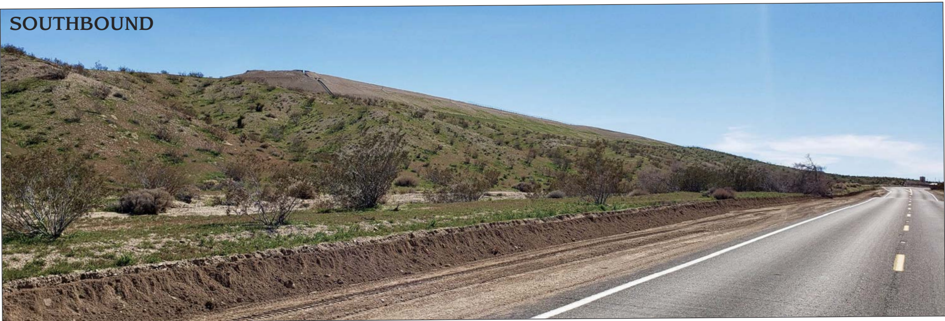
Figure 75SE - Intrusion: The graded slopes of the Barstow Landfill are visible east of the highway, looking southeast at PM 75.
