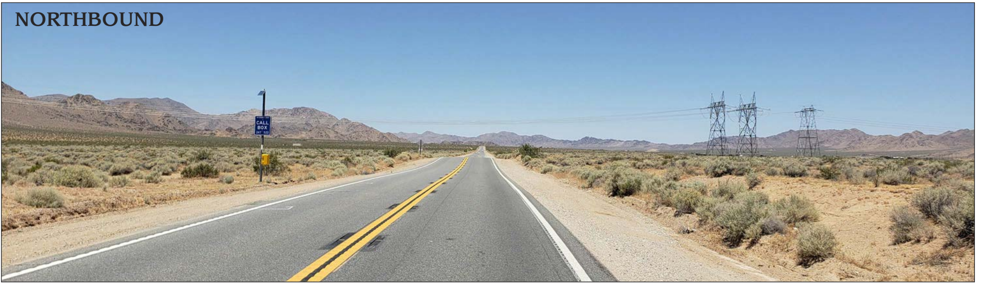
Figure 52N - Intrusion: The three parallel SCE transmission lines cross the highway just north of PM 52.
