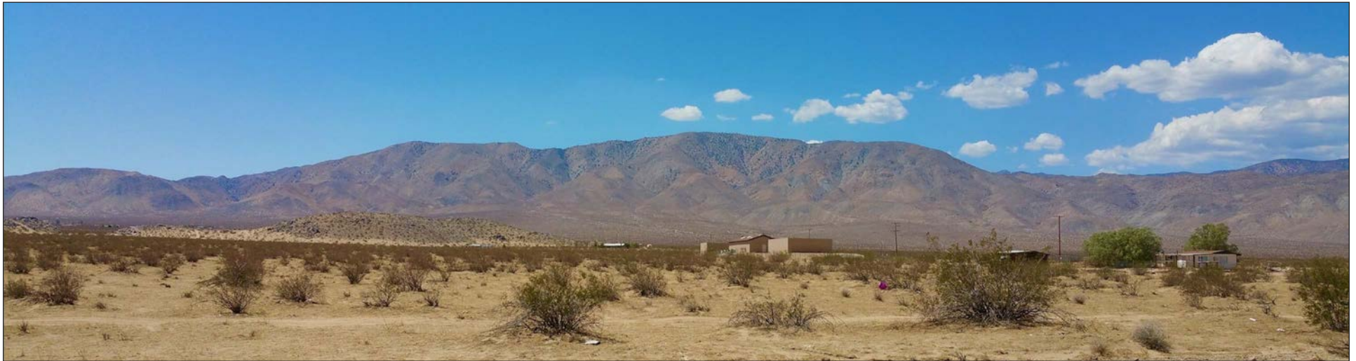
Figure 24.1S - Intrusions: Looking south to the pump station and adjacent homes on Pony Road near PM 24.
