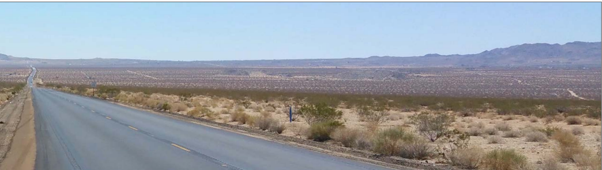
On the far right in the photo one can see the old county route, abandoned when the highway was realigned and paved in the mid-fifties.
