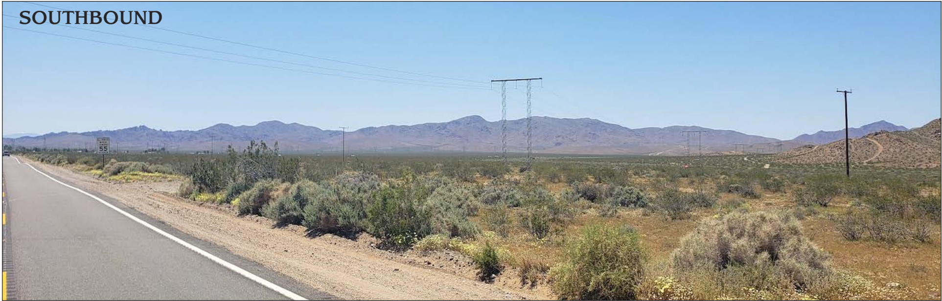
Figure 70.4SW - Intrusion: Transmission line crosses SR 247 at PM 70.4.
