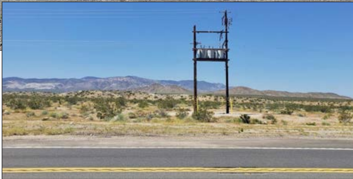
PM 31.3W - Scenic View with Intrusion: A transformer on the west side of the highway, seen from PM 31.3 looking west.
