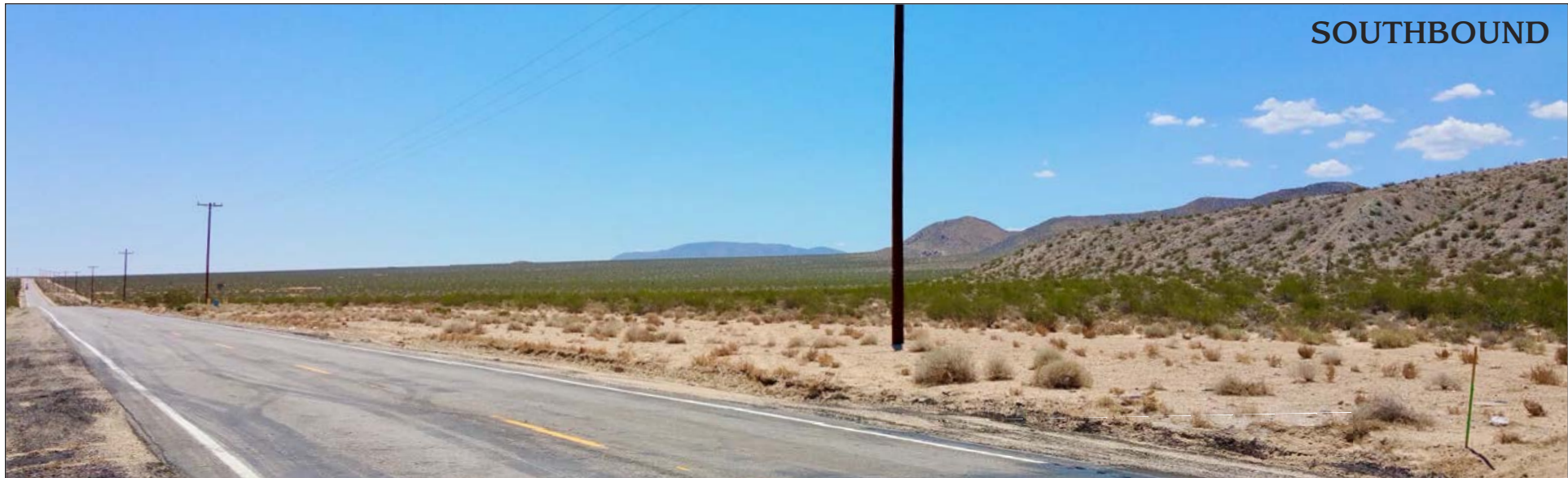
Figure 35E - Scenic View: The toe of the Blackhawk Landslide as seen by the southbound traveler looking south at PM 35. At the center of the photograph is Bighorn Mountain, seen at a distance of thirteen miles.
