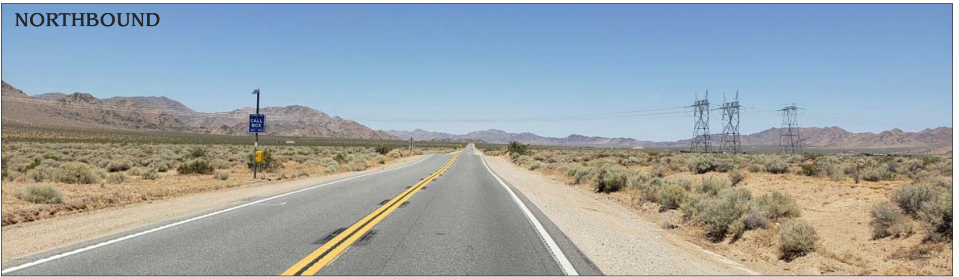
Figure 52N - Intrusion: The three parallel SCE transmission lines cross the highway just north of PM 52.
