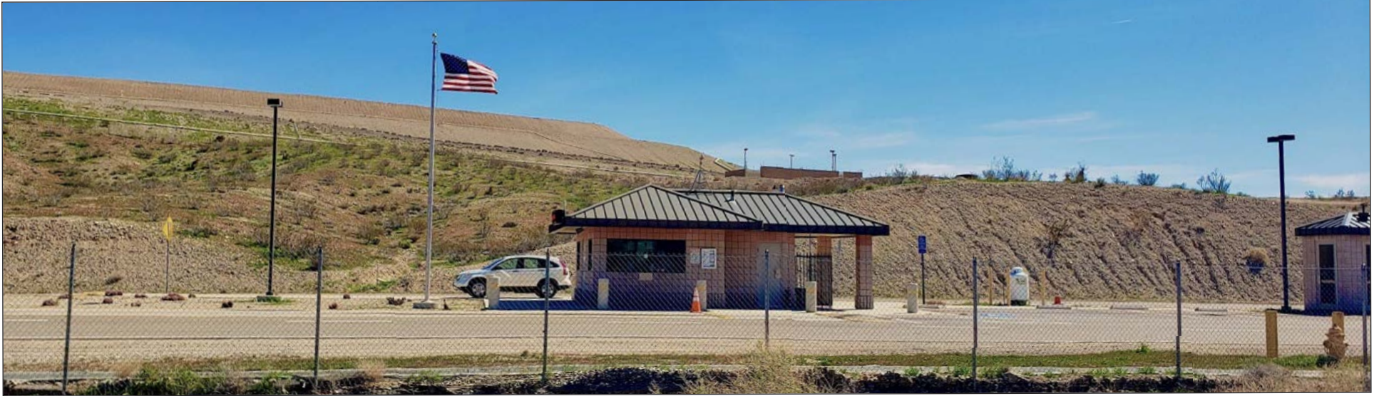
Figure 74.5E - Intrusion: The entry to the Barstow Landfill sits on the east side of the highway near PM 74.5.
